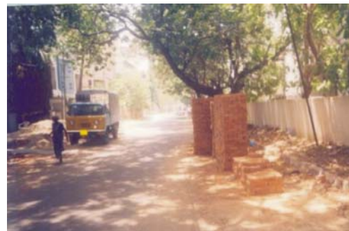
Fig. 28. Dumping of Building materials
