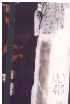
Fig. 14. Failure Mode of S4C Specimen
